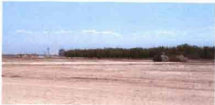
Removing Top Soil from Swall Basin's Site #1
